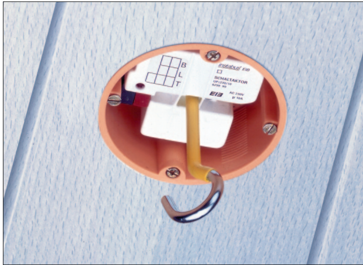
Fig. 2.5-9 Flush-mounted switching actuator in a ceiling socket
